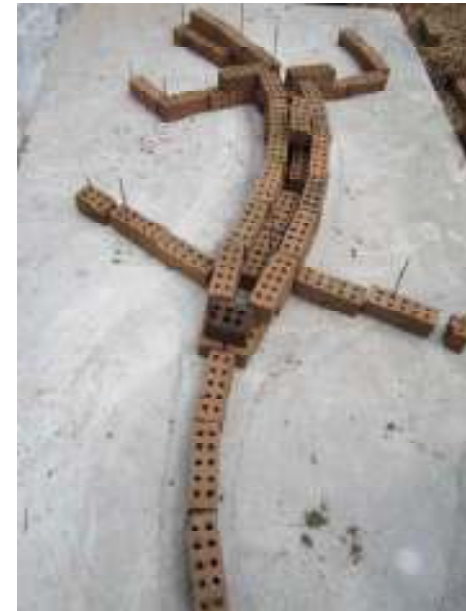
Placing bricks to height of Pins less 5cm
