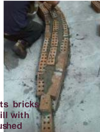
Placing bricks to height of Pins less 5cm
