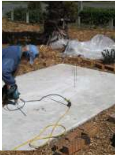
Mr Philips drills holes for steel stakes
