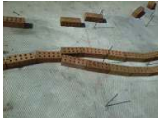
Chicken wire goes under bricks, over pins
