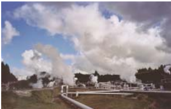
Wairakei geothermal power station.
