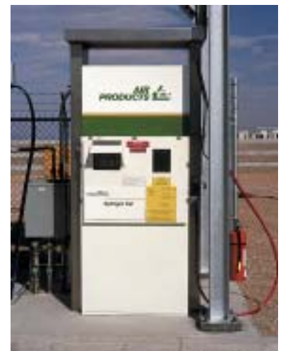
1 Hydrogen fueling dispenser at the Las Vegas Energy Station
