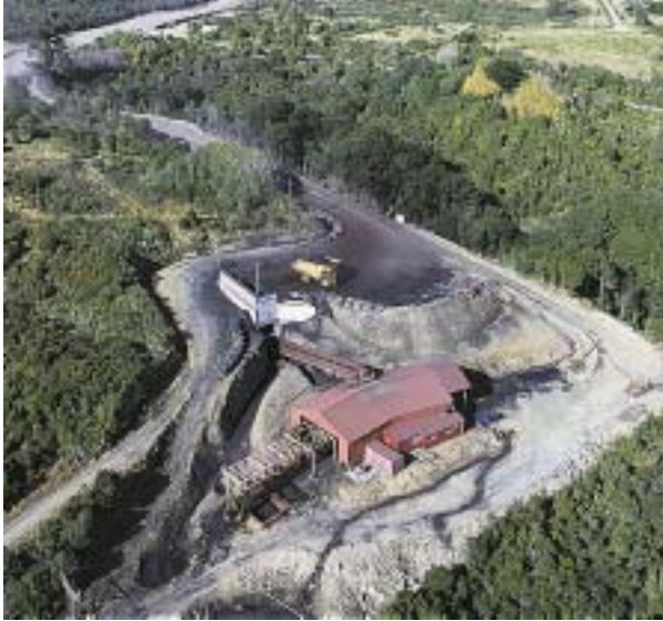
Millerton coal infeed near Westport. Photo courtesy of SolidEnergy
