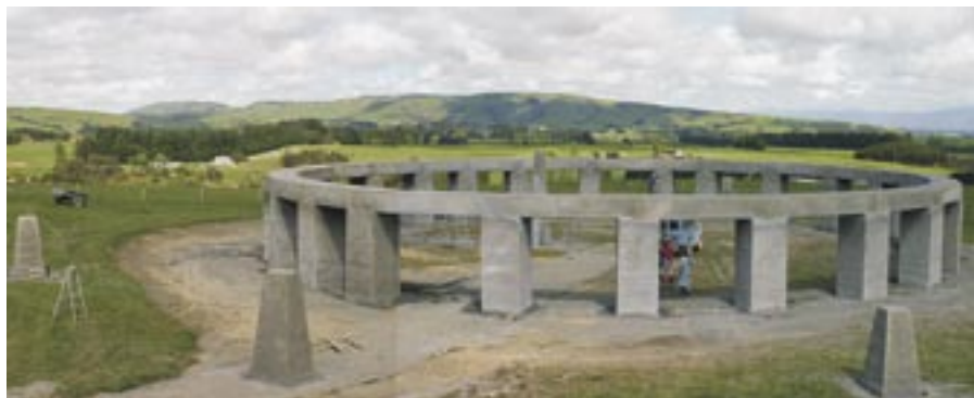
Stonehenge Aotearoa under construction. Photography by Chris Picking.
