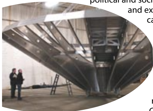
↑ A prototype 12 metre radio telescope under construction in Auckland.
